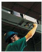
When compared to pipe and wire, busway is an easier to install solution that does not require specialized labor or tools.
