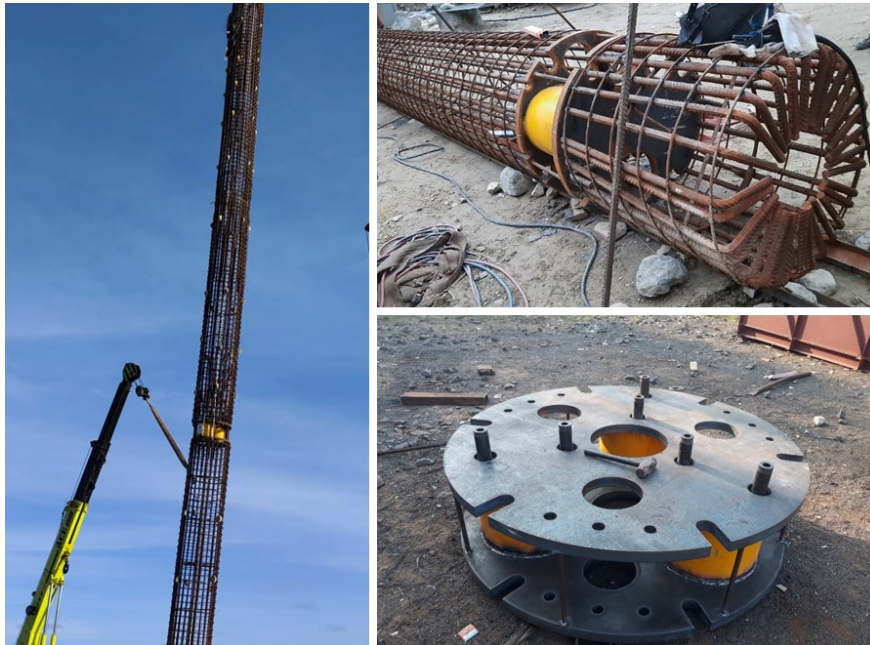
Figure 4: BDSLT setup; Picture Courtesy: GEO DYNAMICS
