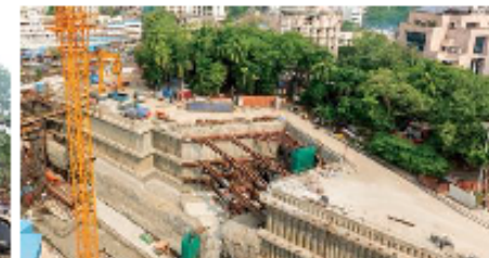
Secant Piling in Mumbai
