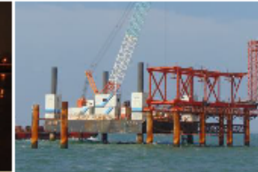
Marine RCD Piling—Udangudi
