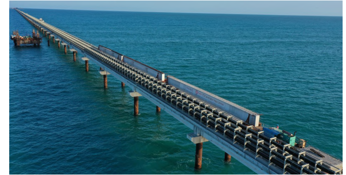
Fig. 4: View of Approach Bridge
