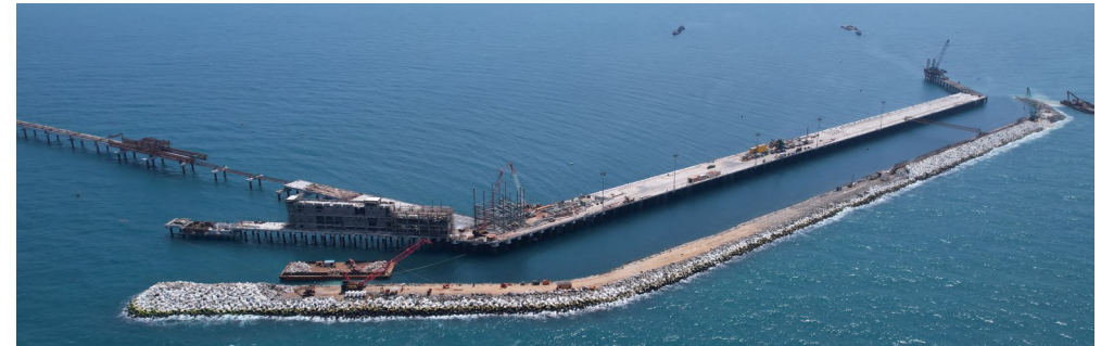
Fig. 2 View of Coal Jetty & Breakwater
