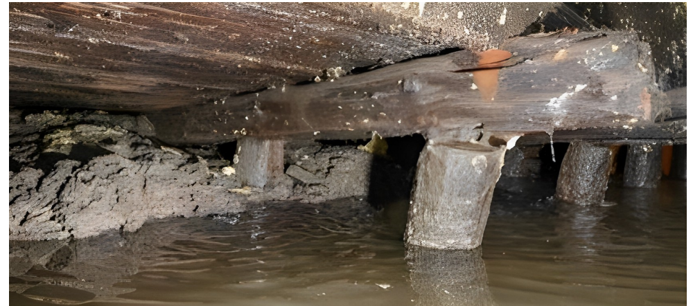
Fig. 1: Timber Piles of the Foundation
