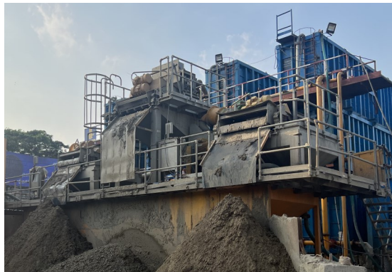
Fig. 3. Desanding plant (Pic Courtesy: Bauer Engineering India)
