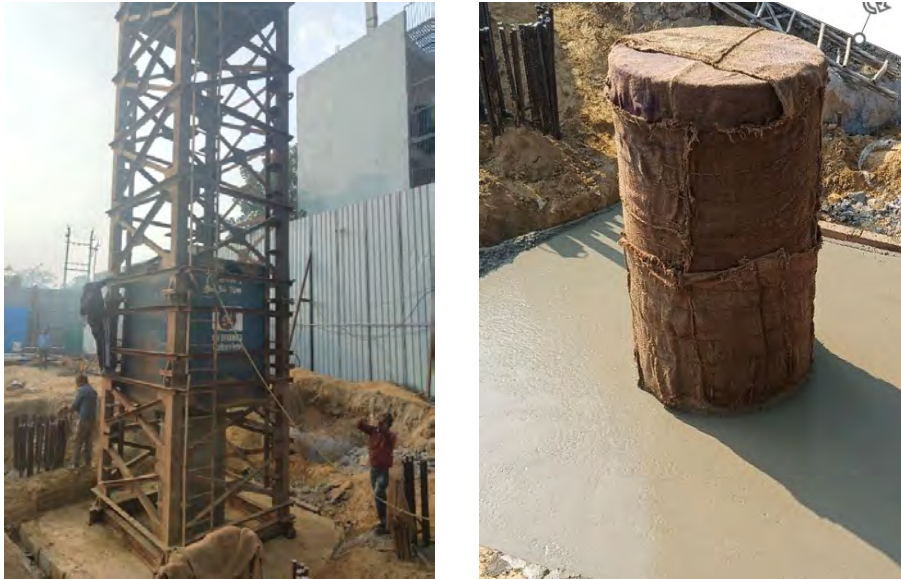
Fig. 1: Typical Guide System and Hammer for Conducting HSDT (Geo Dynamics)
