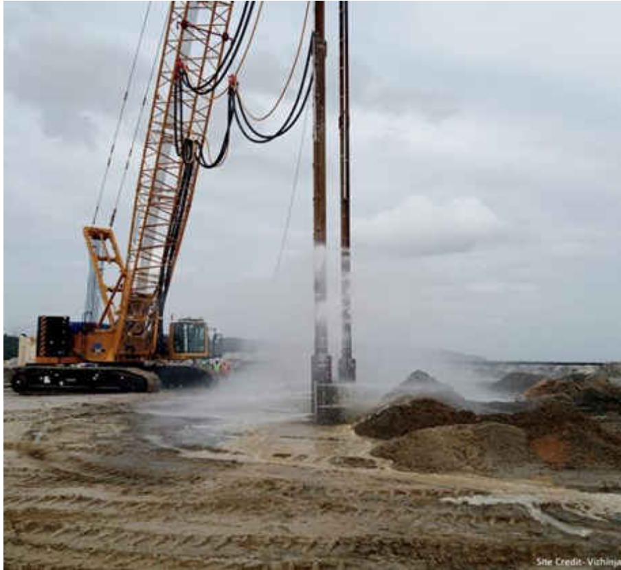
Vibrocompaction with tandem vibrating probes and water jetting for Deep Ground Improvement
