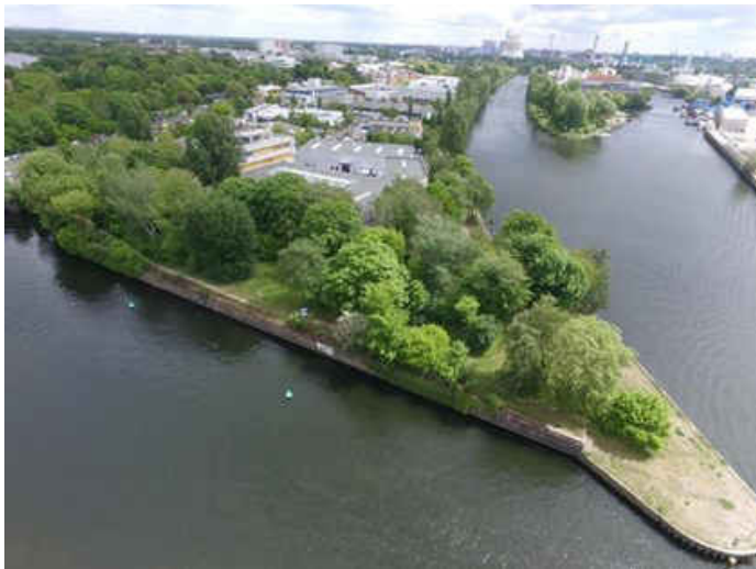
Fig. 1: Steel sheet piles employed in the Charlottenburg Canal – Germany© WNA-Berlin
