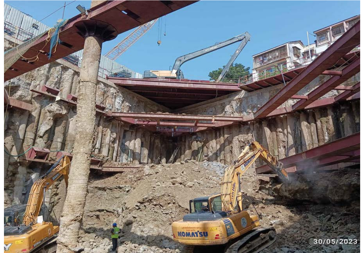
Excavation for Raft Foundation (3000mm), excavation depth 18300mm & Supporting system (Waler beams/Struts & Rock Anchoring) – Girgaon (Mumbai)
