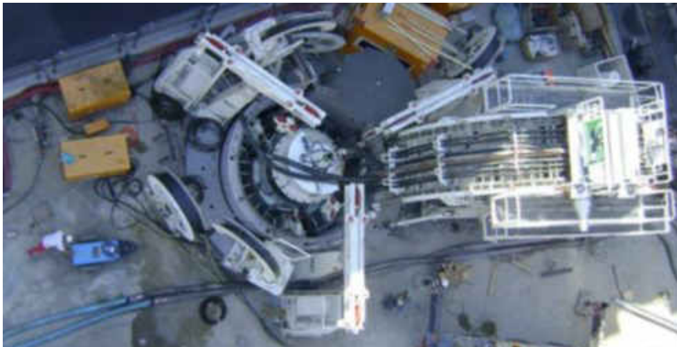
Fig. 4: VSM construction in Naples
