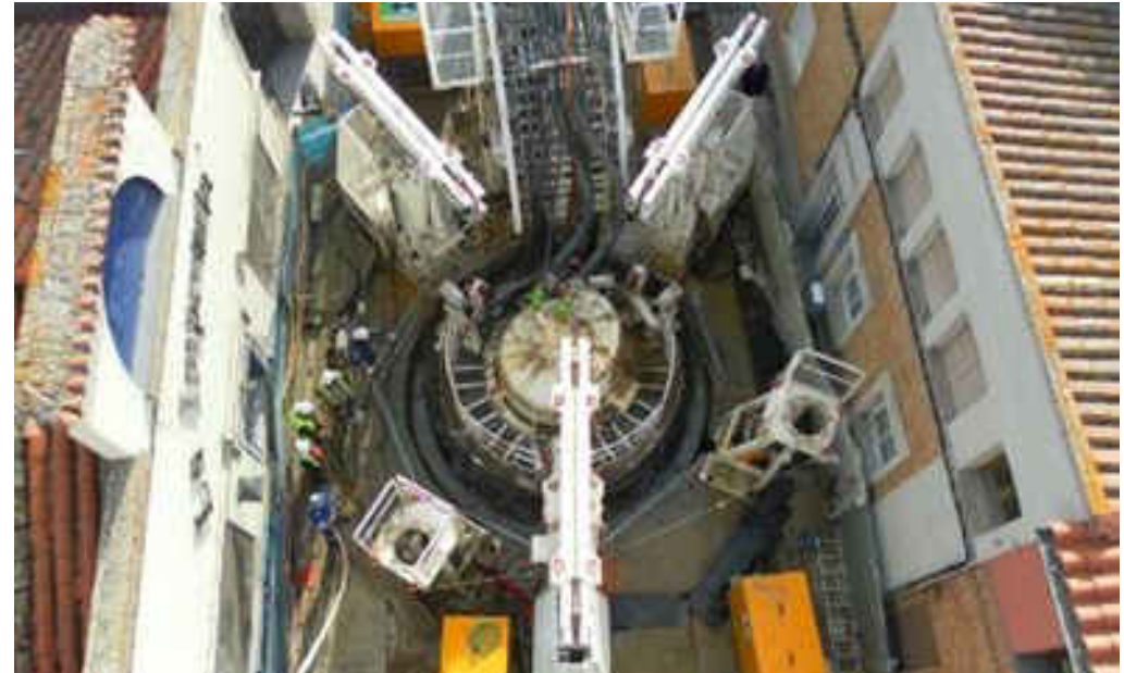
Fig. 5: VSM ventilation shaft in Barcelona
