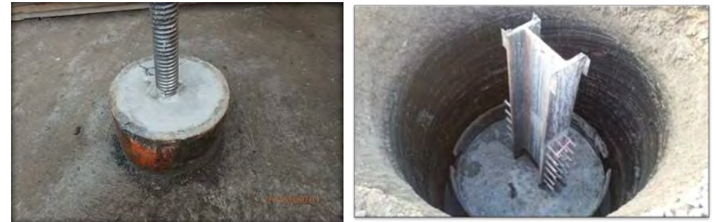
Fig. 2: Typical Caisson Pile Conditions at Pile Cut-off
