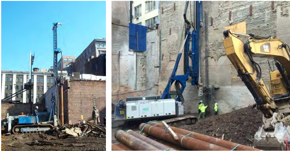
Fig. 3: Typical Caisson Pile Rigs
