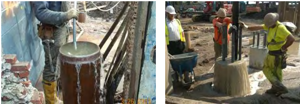
Fig. 6: Flushing of Casing and Rock Socket and Tremie-Grout/Concrete placement
