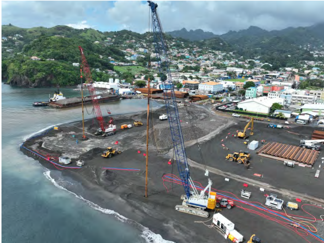
Ground Improvement in Kingstown's Port Modernization in Saint Vincent and the Grenadines
