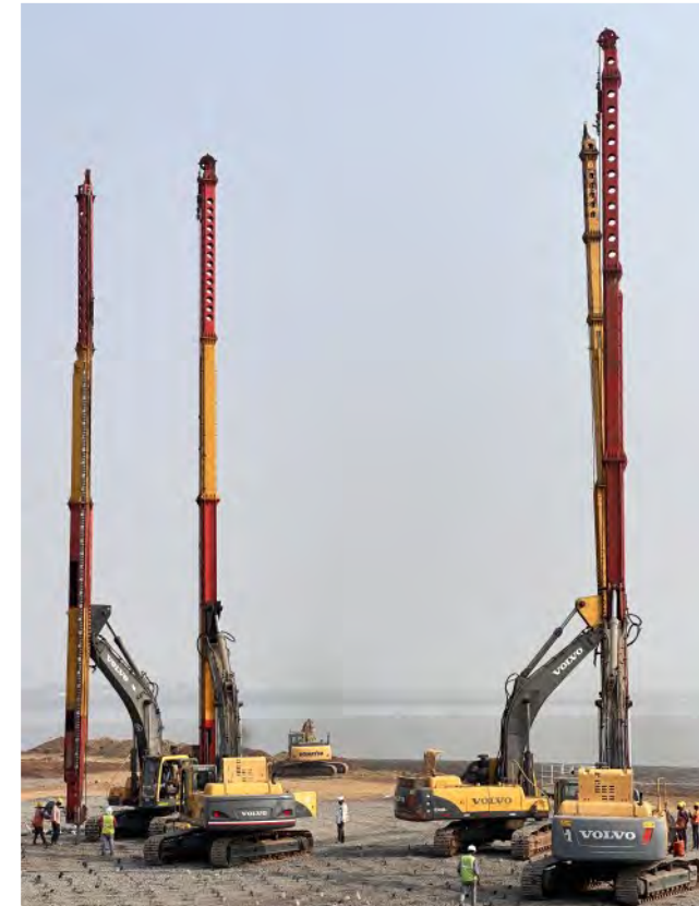
Ground Improvement by Installation of PVD at JNPT Area in Mumbai
