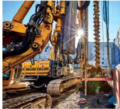
Fig.3: MIP by executing a retaining wall for an excavation pit in Germany
