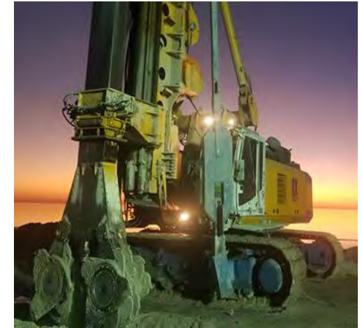
Fig. 6: CSM by executing a Cutoff wall in Canada (Diavik)
