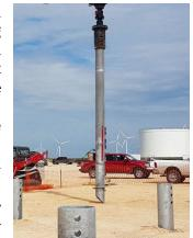
Fig. 1: Helical Pile
