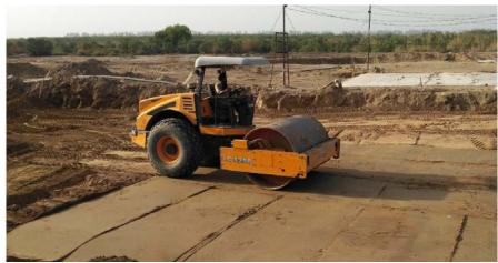
Fig. 1: Soil-Cement Stabilization Ground Improvement Method
