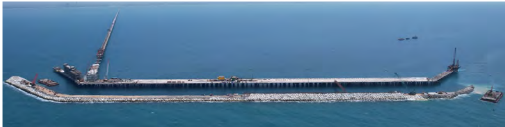
Fig. 1 Island Breakwater and Coal Jetty - 8 km away from the shore
