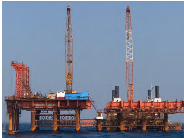
Fig. 3: Pile installation work at Berth Location
