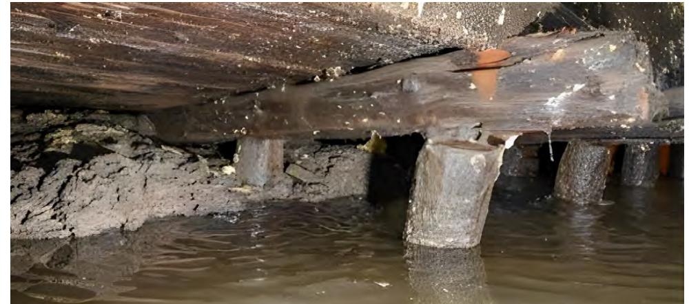
Fig. 1: Timber Piles of the Foundation
