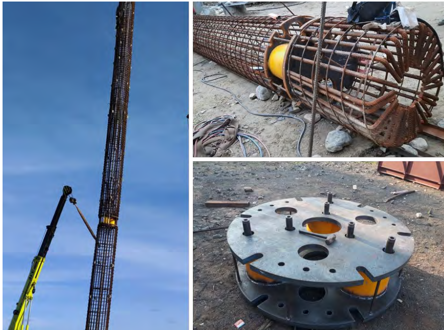
Figure 4: BDSLT setup; Picture Courtesy: gd GEO DYNAMICS
