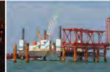
Marine RCD Piling—Udangudi
