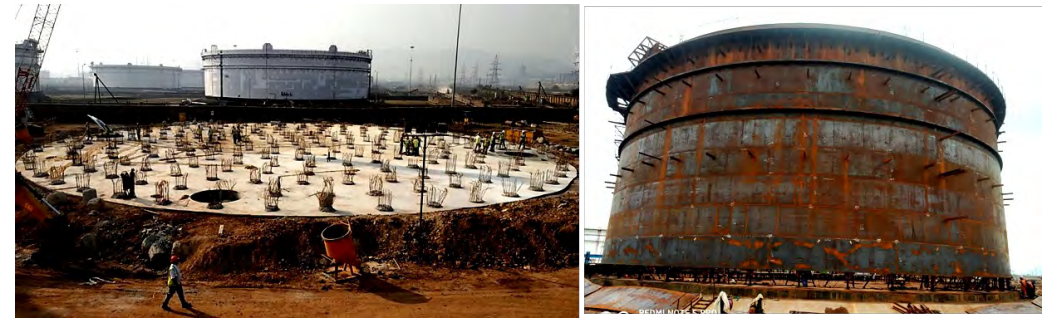
Fig.1. Pile cap connecting the installed piles and tank erected on the foundation
