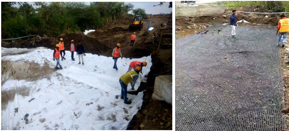
Fig 3 and 4: Laying of non-woven geotextile, Laying of woven polyester geogrid
