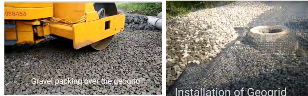
Fig 5 and 6: Laying of Biaxial geogrid towards the topmost layer, Gravel packing over the bi-axial geogrid.
