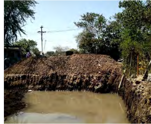
Fig 1. Accumulation of water at the approach road location
