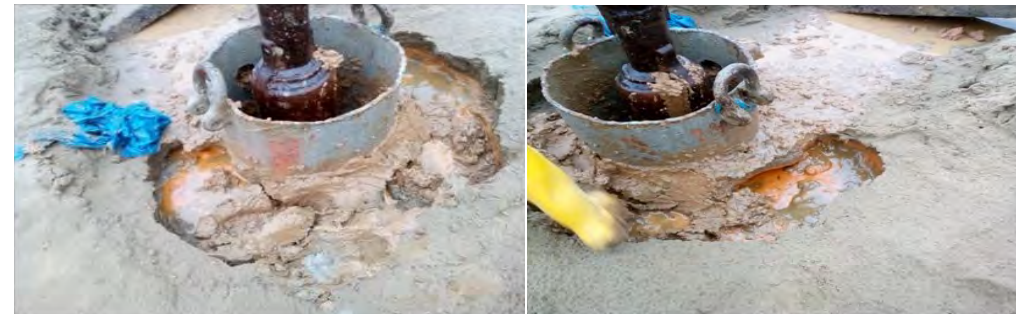
Fig. 2. The condition of the bore round liner (liners where installed with pre-bored holes of higher dia.)
