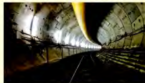
India's first underwater Metro tunnels under Hooghly River, Kolkata using 6.55m dia TBM completed in just 67 days
