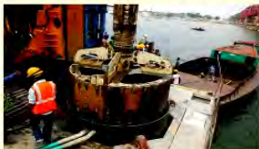
Use of 2.5m dia, 68m deep concrete piles for second Bhairabgarh Bridge across Meghna River in Bangladesh
