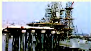
One of the longest jetties (2.5km) founded on driven steel piles at Hazira in Gujarat
