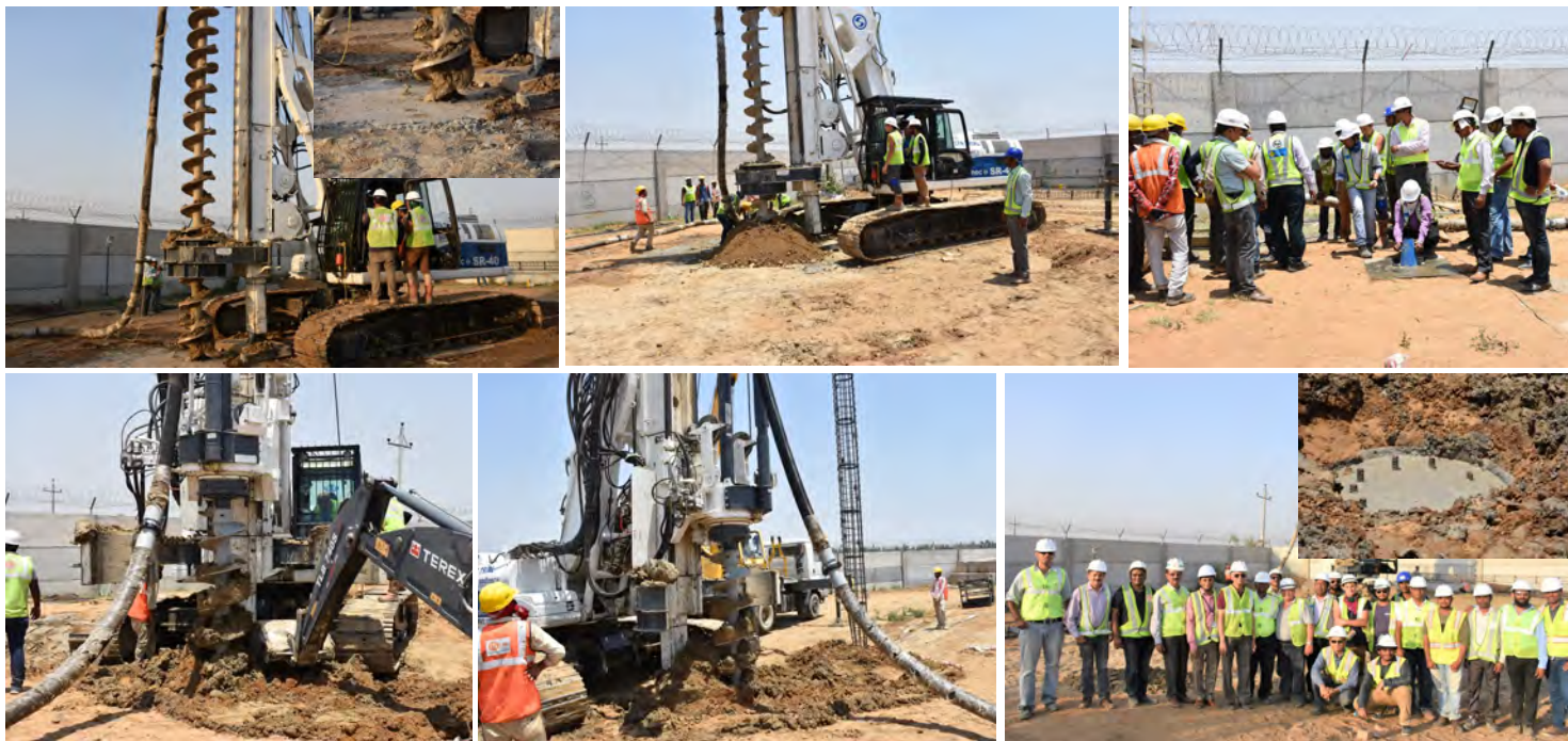
CFA trial Pile installation photos at NPCIL Site, Hisar, Haryana during various stages of installation
