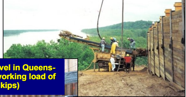
SBMA into loess silt at Natchez, Mississippi, test loads of 890kN (200 kips)
