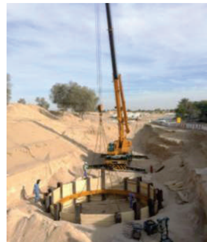
Pic. 5: View of a circular waling being installed in Manhole No. 73 at Al Khawaneej Project Site
