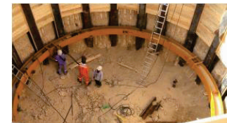
Pic 3: View of a typical circular waling with three segments and three connectors
