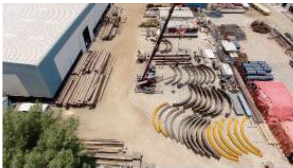
Pic. 6: Ariel view of ESC Yard where circular walings are being fabricated for Al Khawaneej Project Site
