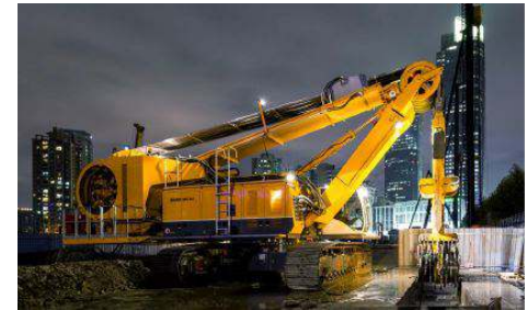
Figure 3: Wire rope-suspended CSM unit, China.
