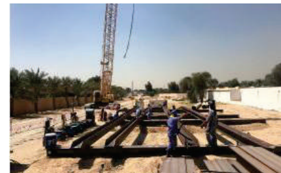
Pic. 4: View of a set-up for kingpost fabrication at Al Khawaneej Project Site
