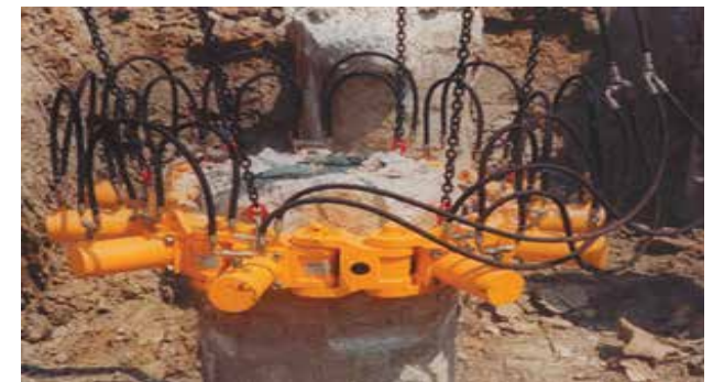
Fig. 4: Hydraulic Pile Head Breaker
