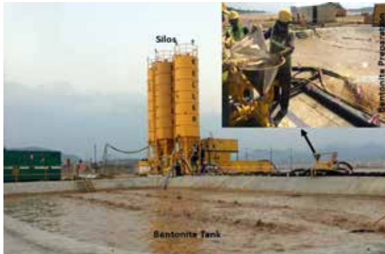
Fig. 5. Batching and mixing setup
