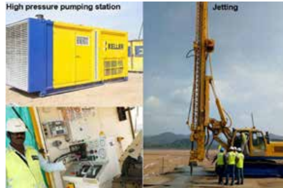
Fig. 6. High-pressure pumping and jetting setup
