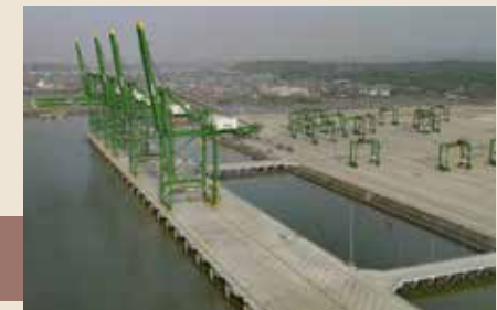
India's largest container terminal founded on bored cast in-situ concrete piles; completed in record time at JNPT
