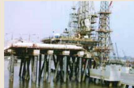
Use of 2.5m dia, 68m deep concrete piles for second Bhairabgarh Bridge across Meghna River in Bangladesh
