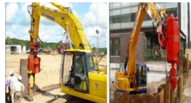
Fig. 5: Side Grip Vibro-cum-Impact Hammer System for Sheet Piling
