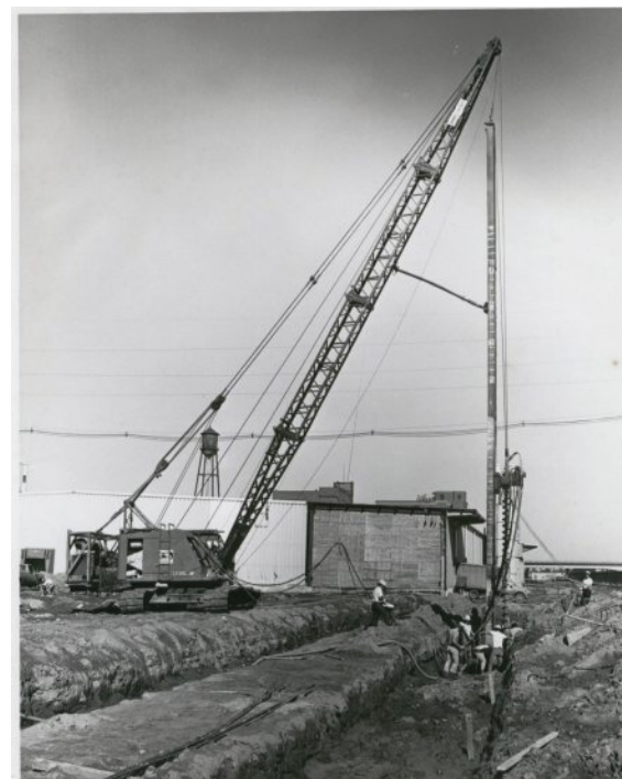
Early installation of ACIP piles
