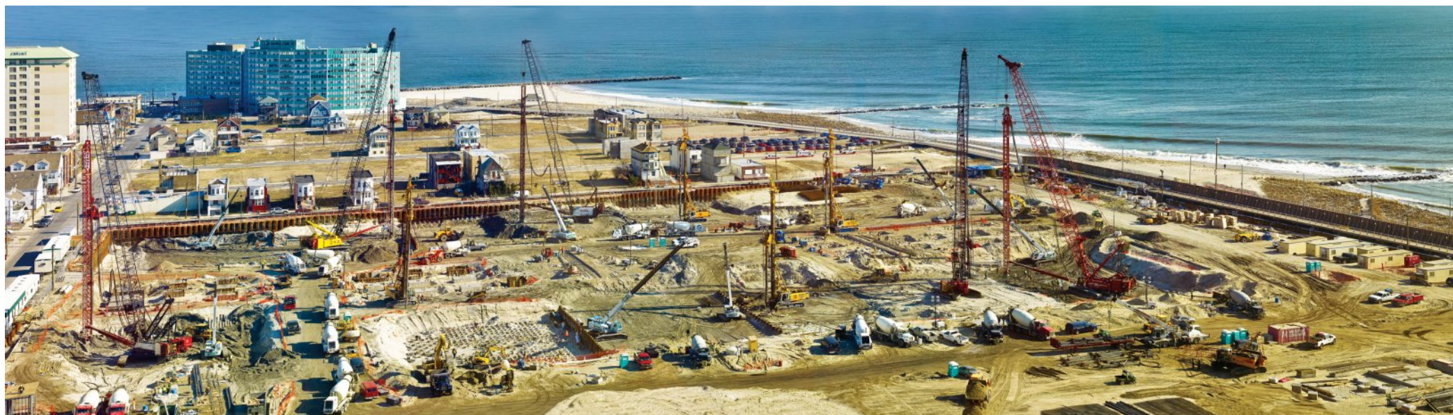
ACIP piles being installed at the Revel Casino in Atlantic City, NJ
