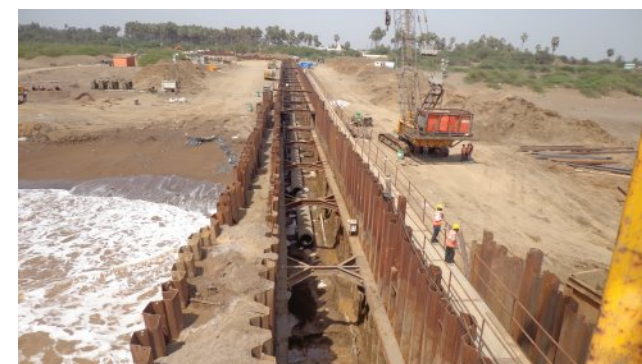
Sheet pile work for laying under-sea LNG pipeline at 5m below ground level at ONGC, Hazira
