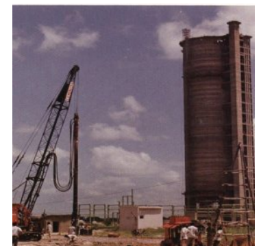
Prilling Tower (106 Meters) at Babrala (UP) resting on Ground Improved with Vibro-Stone Columns
