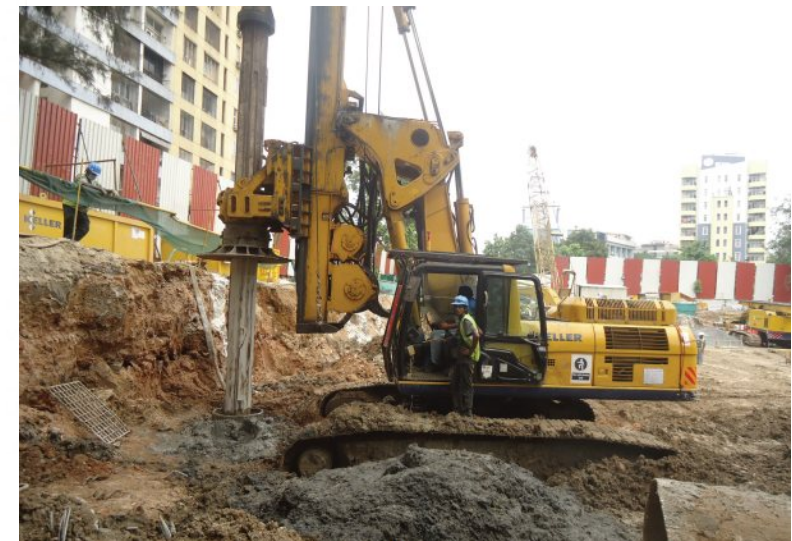
Step 1B: Contiguous Bored Pile Drilling in Progress
