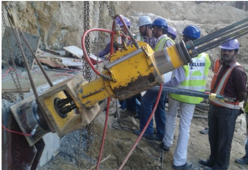
Step 5: Stressing of Anchors
