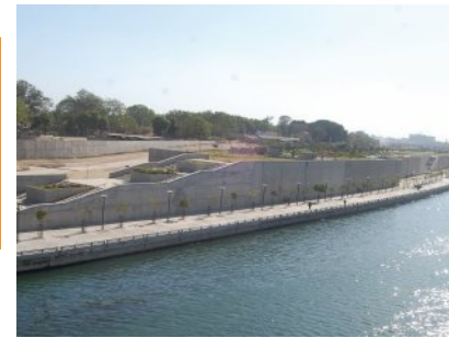
13.5 kms Diaphragm Wall for Sabarmati River Development Project
