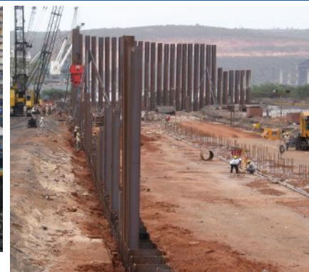
PTC 60HD vibrodriver driving a combined wall made of Arbed HZ975 and AZ18 sheet piles for a new wharf in the harbour of Visakhapatnam. Contractor: Afcons
