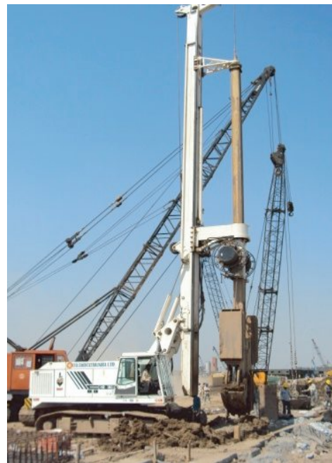
FIG. 5: Kelly operated hydraulic grab
