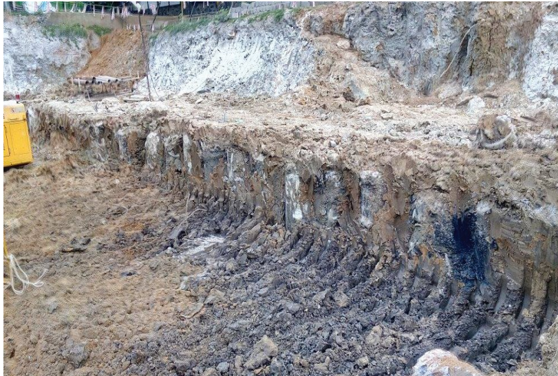
Step 1C: Installed Contiguous Bored Piles
