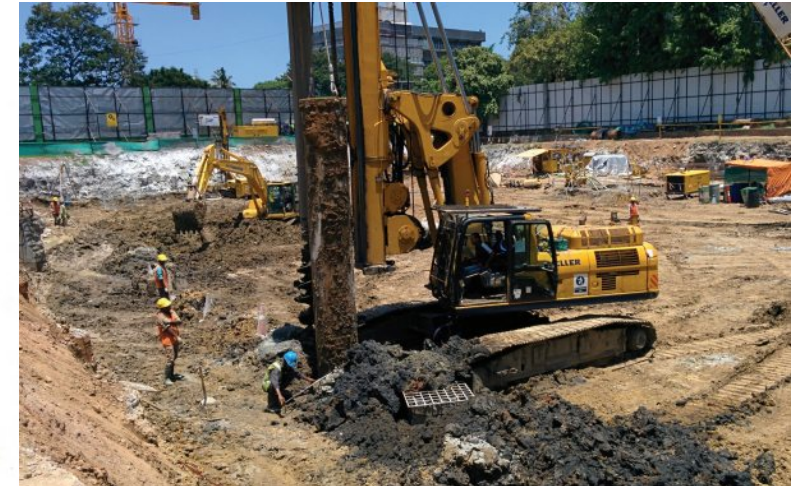
Step 1A: Positioning of Hydraulic Piling Rig & Installation of Temp Casing
