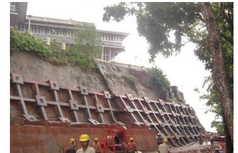
Slope Stabilization at Raj Bhavan, Cabo Hill, Goa
