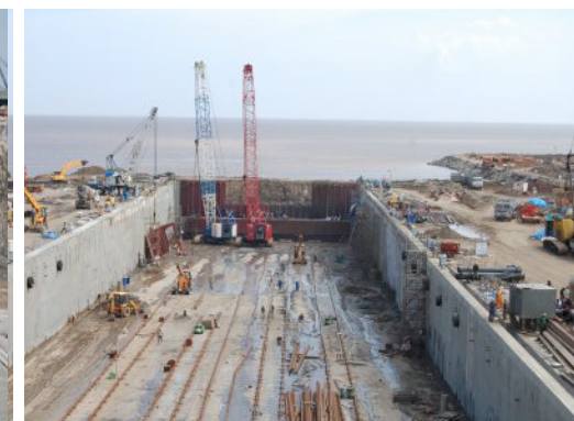
Fig. 8 Completed DW at Slip Dock with Pontoon Gate under Construction
