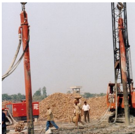
PTC 65HD vibrodriver extracting 29m long HEB300 for the extension of the New Delhi metro. Contractor: Afcons
