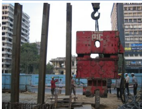
PTC 65HD vibrodriver extracting 29m long HEB300 for the extension of the New Delhi metro. Contractor: Afcons
