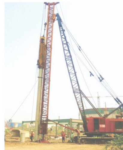
Spun Pile Driving at Dahej, Gujarat
