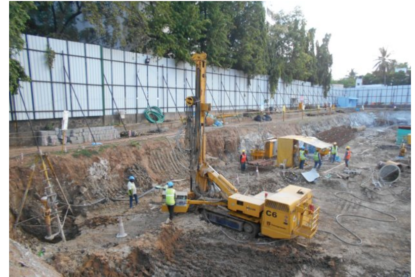
Step 2: Installation of Grout Columns
