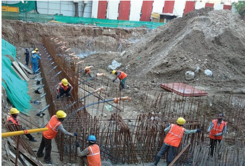
Step 4B: Cage fabrication of Capping beam
