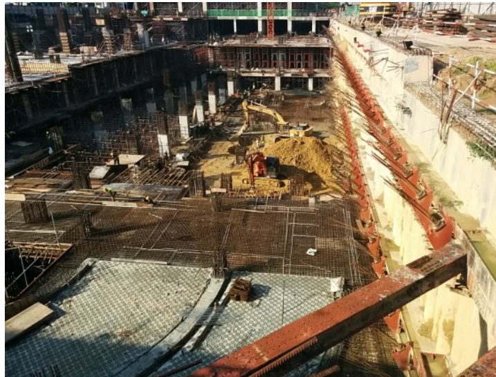
Step 6 Final Excavation
