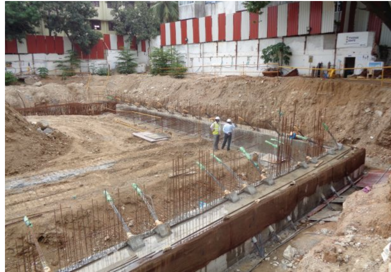
Step 4C: View of Capping Beam after Concreting
