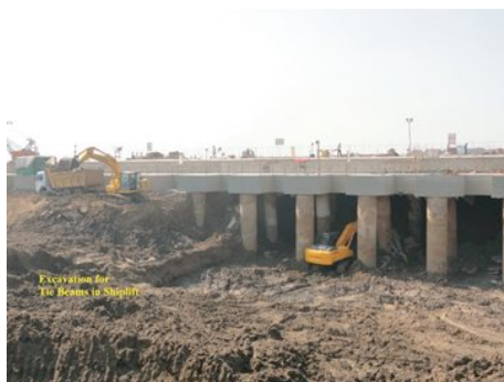
Fig. 4: Excavation at Shiplift area & Exposed Vertical & Raker Piles.
