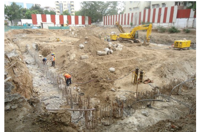
Step 4A: Pile Chipping
