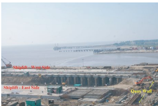
Fig. 3: Piles along Shiplift Facility & Quay Wall Location
