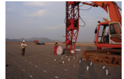
PVDs for Reclamation Works of 4th Container Terminal, JNPT, Mumbai
