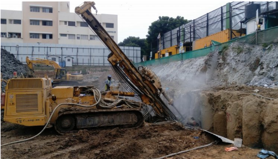
Step 3: Installation of Inclined Soil Anchors
