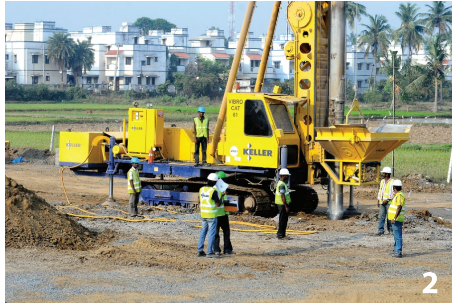
Step 3: Penetration of depth vibrator to required level
