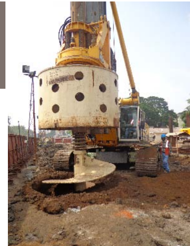
Piles of dia 2500mm and depth 33m in hard rock strata for metro stations in Chennai
