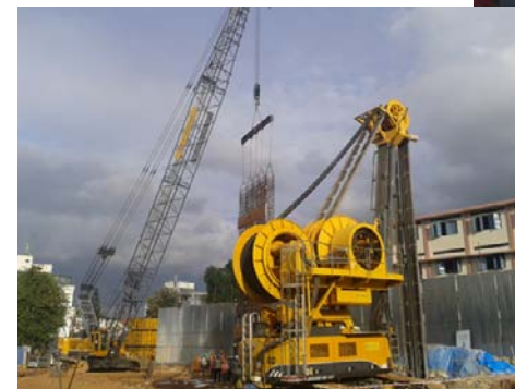
27m deep d'wall on D&B basis, creating 5 basements in Bengaluru
