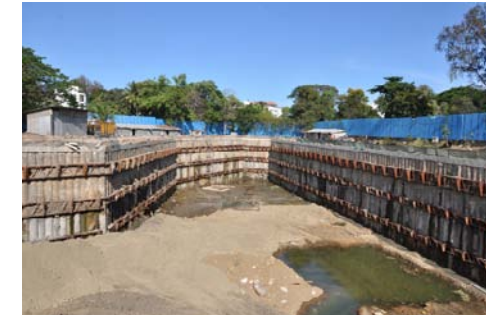
20m deep secant pile walls and 3 levels of anchors at Chennai
