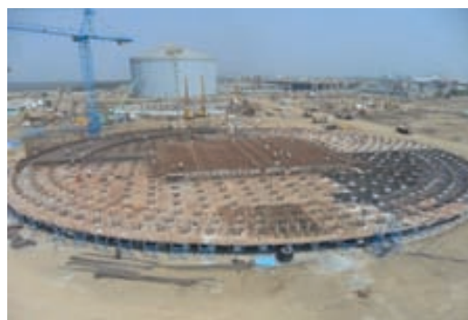
Installation of large diameter Bored Piles for LNG Storage Tanks in Gujarat, India
