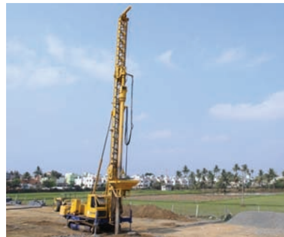
Fig. 4 Installation of Vibro Stone Columns in progress
