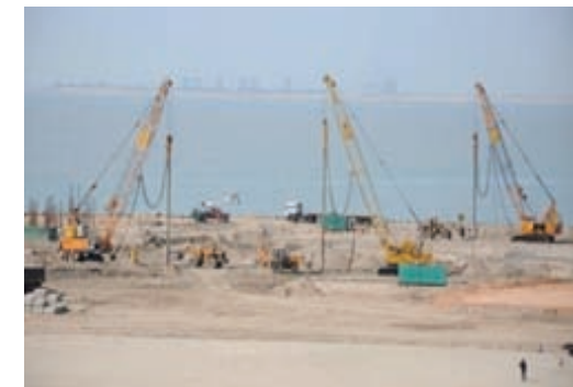
Ground Improvement works (Vibro Compaction & Stone Columns) for LNG Storage Tanks in Gujarat, India
