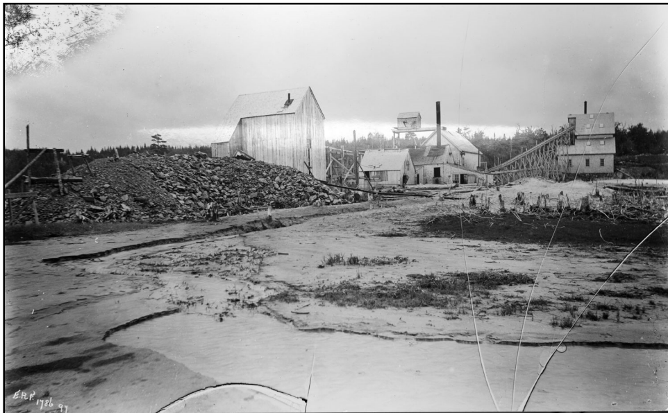
Figure 7. (a) Recovery of Hg amalgam from copper-plated amalgam tables in the 20-stamp mill, Dufferin Gold Mine, Salmon River, Nova Scotia, 1893. The suspended shaking tables below the amalgam plates were used to recover sulfide concentrates (predominantly arsenopyrite). Tailings from each table were discharged from the mill via a wooden trough. (b) Unconfined tailings disposal into the Tangier River from 10-stamp mill at the Mooseland gold mining district in 1897. Photos taken by E.R. Faribault, Geological Survey of Canada and reproduced with permission from NRCan.
