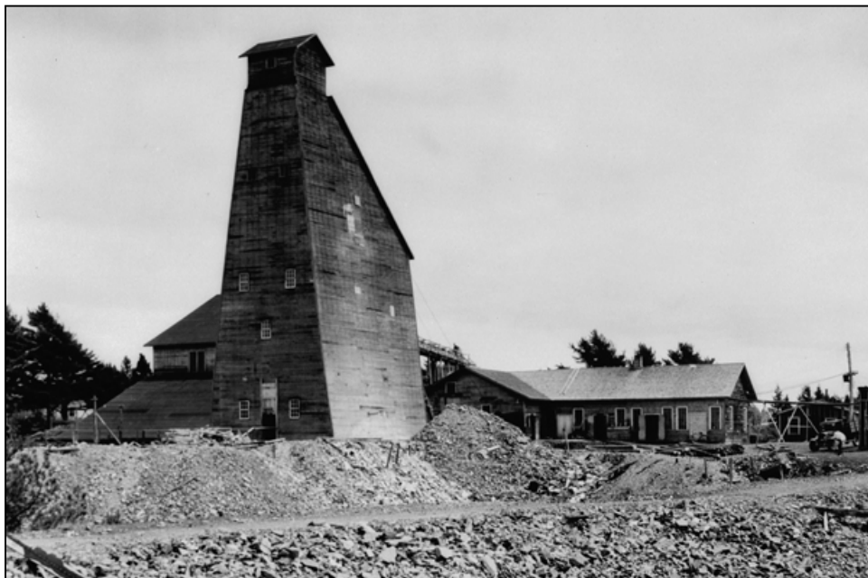
Figure 11. (a) Surface plant showing workings on the Skerry lead, circa 1934. The headframe is the tall building on the far left, and the stamp mill is the peaked building in the distance. The wooden trough emanating from the stamp mill towards the lower left corner of this photo is the tailings launder, which was used to direct the tailings to a downstream wetland on Mitchell Brook. (b) Close-up of the Skerry Shaft headframe with the mine office on the right (Nova Scotia Archives).
