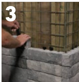
3 Attach Tandem Veneer with Connector
