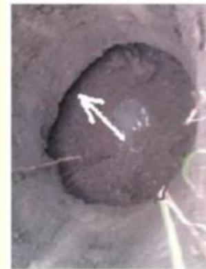
The team learned Whether rain and flood comes in or high ground water it is the bottom soil that softens and results in collapsing the pit. The fact that the collapse is happening from the bottom makes the problem complicated. It is uncommon for collapse to happen from bottom than from the top.
