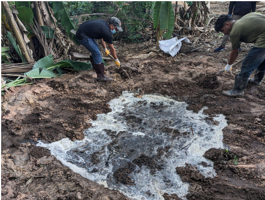
Latrine business workers backfilling the burial pit to prevent treated FS from contaminating the household surface.
