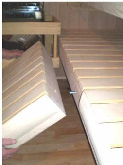
Step 11: Line up the predrilled holes in the bottom bench with the middle platform bench and attach using lag bolts (provided).
