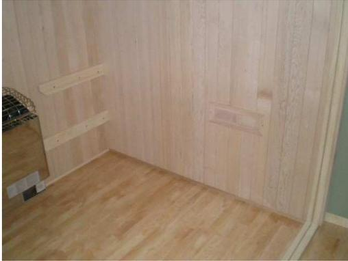
Step 1: Prior to installing the all-glass front, start on the right side of the room and note that the bench supports on the back wall have been pre-installed.
