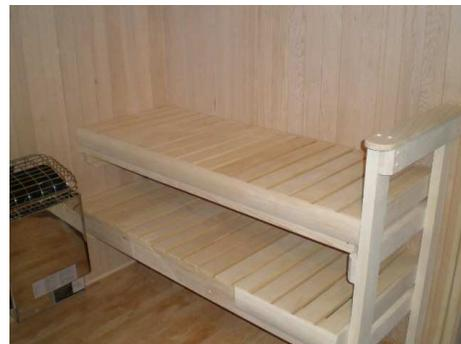
Step 6: Place the top bench on the supports as you did with the bottom bench and secure in a similar manner as the bottom bench. Note the partial bullnose molding on the bottom bench as noted earlier in Step 3.
