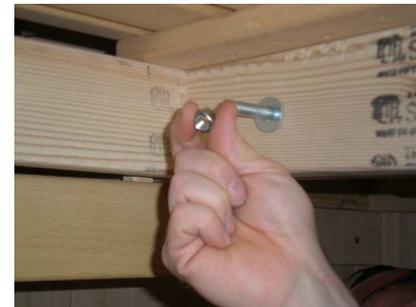
Step 12: Tighten lag bolts to assure rigid bench strength.
