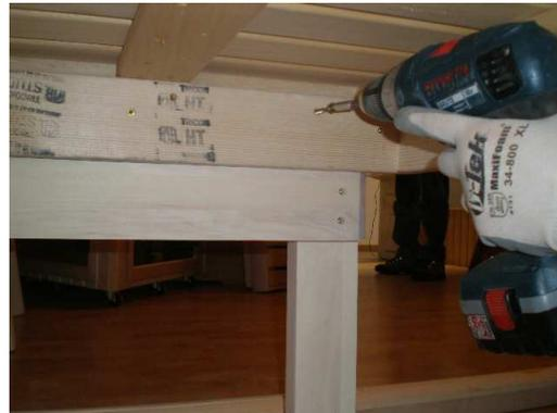
Step 4: Using 2" torx screws (provided), secure the bench to the arm rest assembly. Do this from underneath as shown above.
