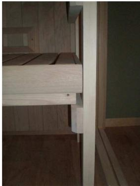
Step 3: Place the lower bench on the back wall support and the lower bench support of the arm rest. Make sure that the decorative bull nose molding is on the front half of the bottom bench. Note that the bottom framework of the bench will rest on the support which will create a small gap between the arm rest and the bottom framing of the bench.
