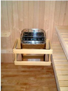
Step 9: Install heater guard around heater making sure that it is evenly spaced around the heater and not touching the heater directly.
