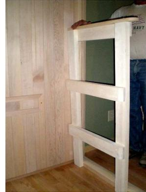
Step 2: Find the free standing (already assembled) arm rest assembly. Make sure that the rounded handle points inward and the ladder supports of the arm rest face inward toward the room.
