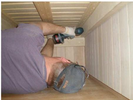
Step 5: Using 2" torx screws (provided), secure the bench to the back wall. Do this from underneath as shown above.
