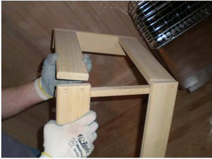
Step 7: Assemble the heater guard with 1 1/2" screws provided according to predrilled holes
