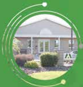
Miller Weldmaster Corporate Headquarters Navarre, Ohio
