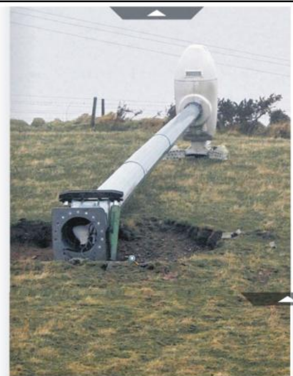
BROKEN: The collapsed wind turbine at Ardiffery Mains yesterday
