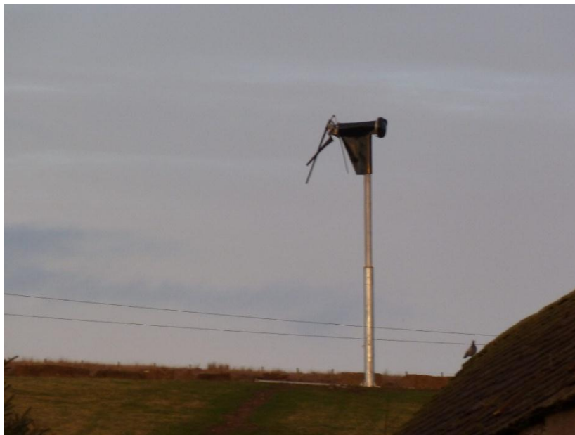
Photograph of a severely damaged turbine taken at Oust in Caithness in January 2013
