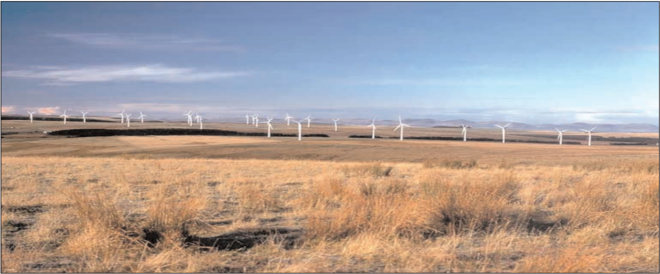
A view of Dun Law power station, near Edinburgh. An extension to the site is under consideration.
