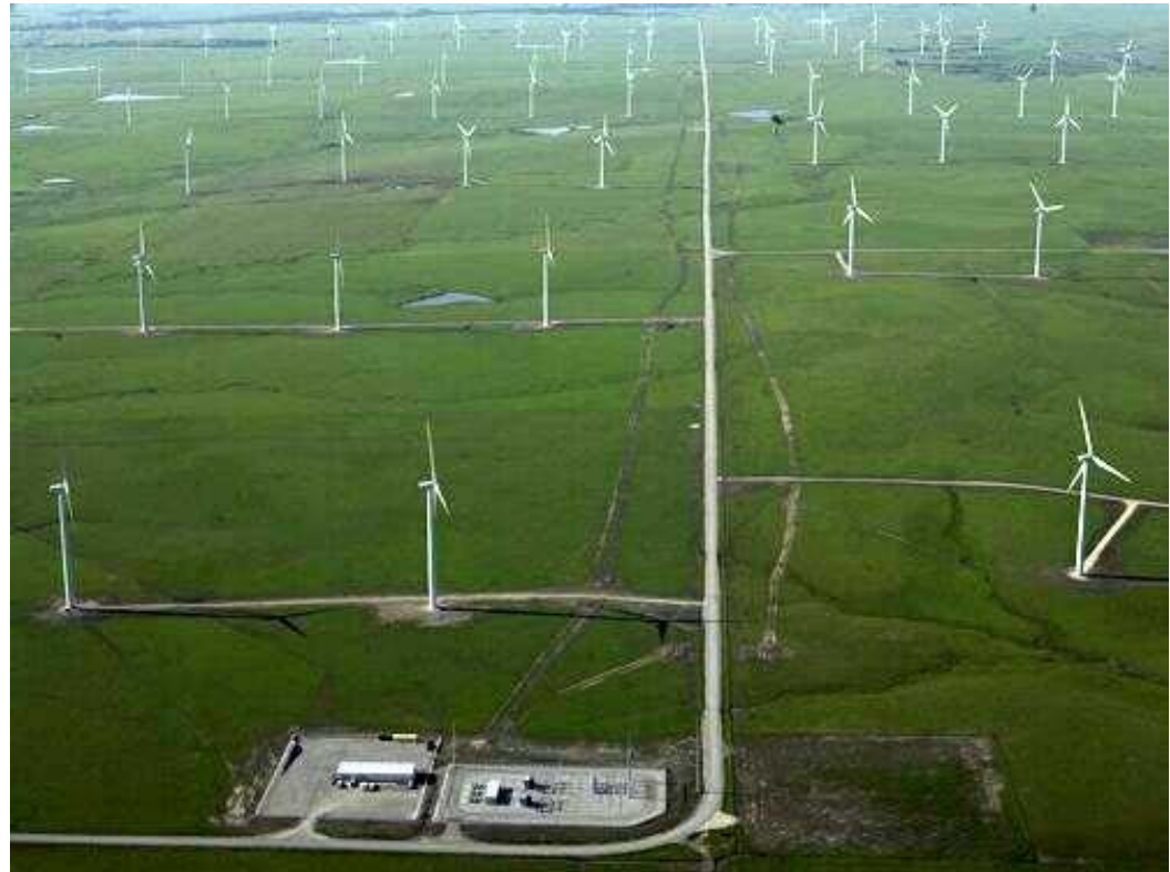
Image: Elk River 150mw facility, Butler County Kansas
