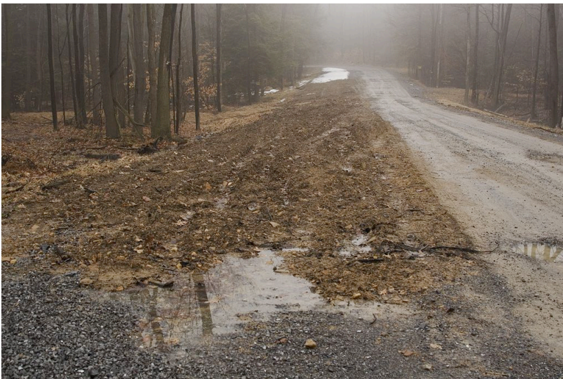
Soil that was spread on top of the gravel along this section of the road is eroding away.
