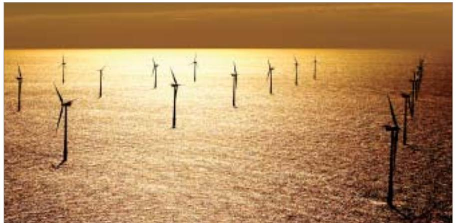
Fig. 1. Completed in December 2003, Nysted offshore wind farm in Denmark has 72 turbines with a total capacity of 166 MW, making it the world's largest (courtesy Elsam)
