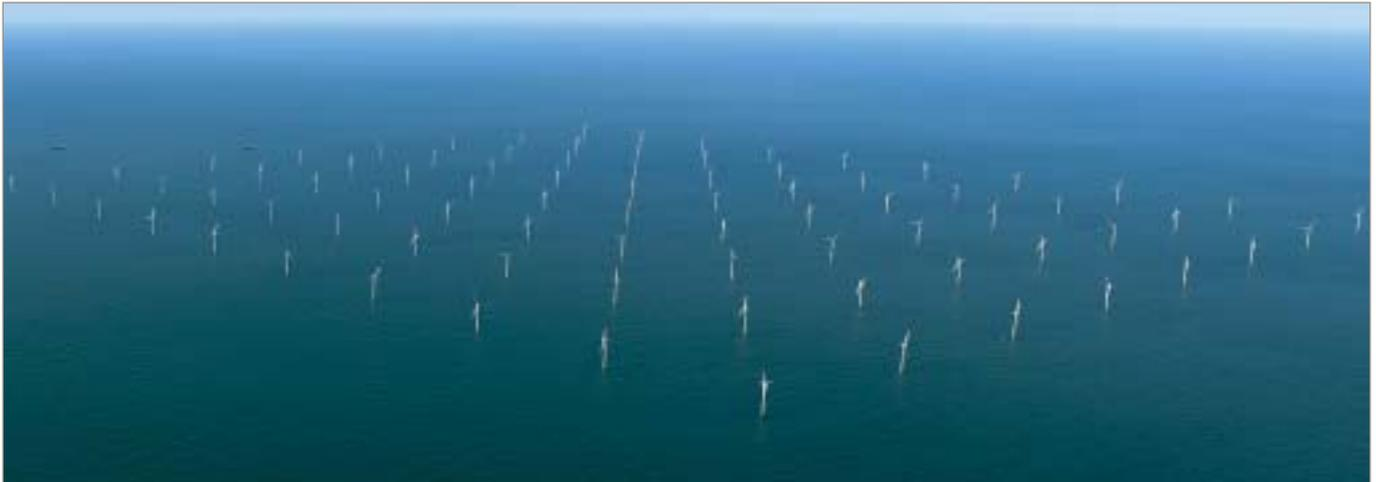
Fig. 4. Horns Rev wind farm has 80 turbines generating 160 MW (courtesy Elsam)
