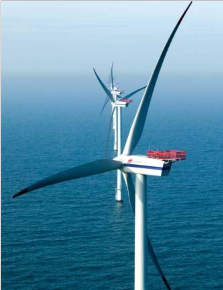
Fig. 10. The Vestas V80 2 MW turbines at Horns Rev need 4 m/s wind speed before they can begin generating but must feather their blades at around 25 m/s to prevent mechanical damage
