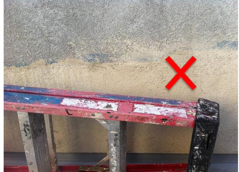
*Notice the paint and grime covering the labels and steps of this ladder. It should be removed from service and cleaned to avoid a potential safety hazard. (\*8)*
