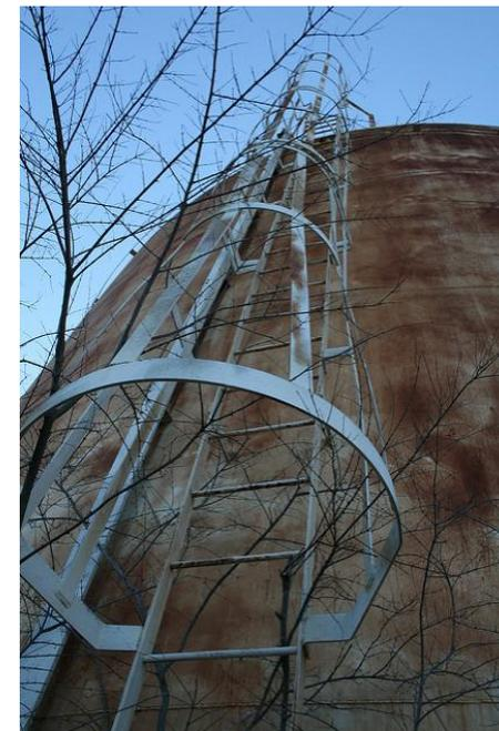
Inspect fixed ladders for missing rungs, bolts, burrs, or other deformities before use. (\*5)
