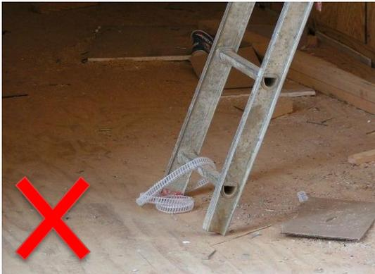
*Extension ladder missing foot pads and foot assembly. This appears to be the top portion of an extension ladder that has been taken apart.*
