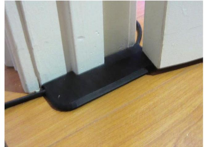
Extension cord under door with a protective device to avoid potential damages. (\*4)
