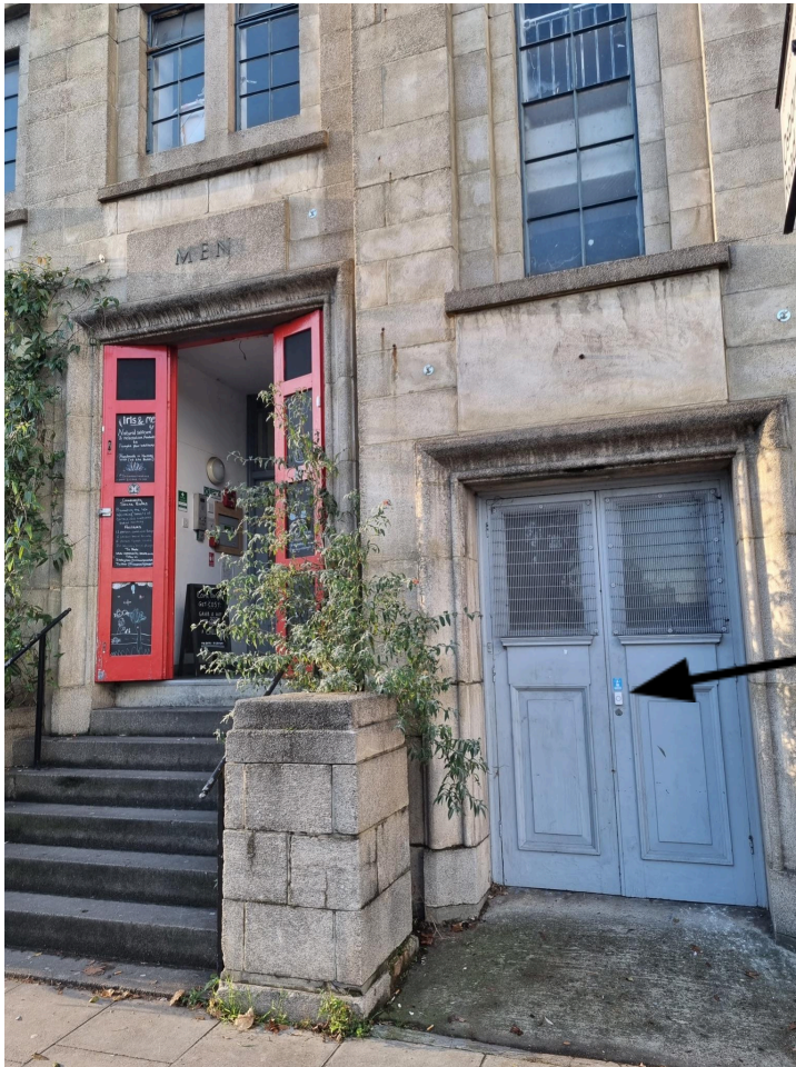
Grey door to platform lift next to main entrance (arrow pointing to doorbell)
