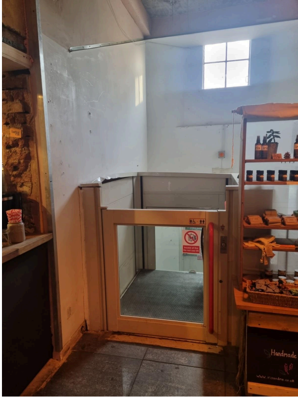
Platform lift from café to Eastway entrance
