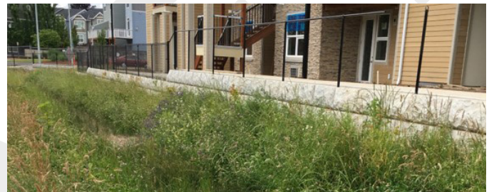
Stormwater planters filter runoff and create a pleasant transition
