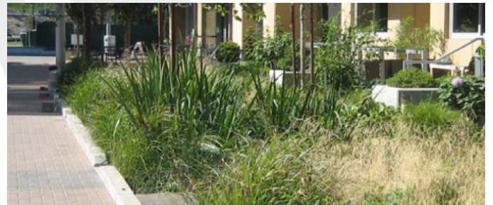
Bioswales in a residential development treat stormwater runoff
