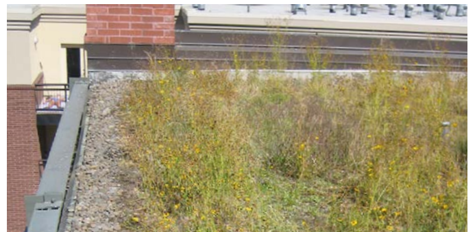
Ecoroofs should be incorporated in building design whenever possible
