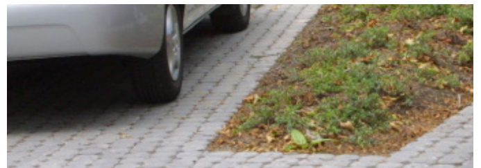
Sustainable design through permeable parking surfaces
