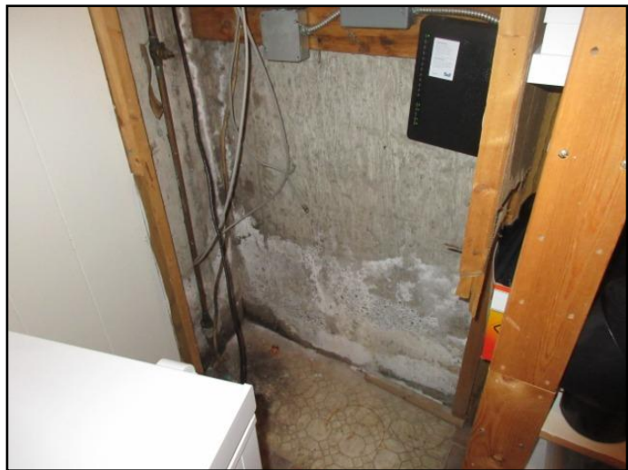
25. Efflorescence
