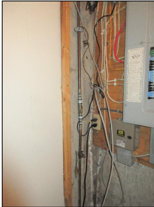
18. Main water shut off
