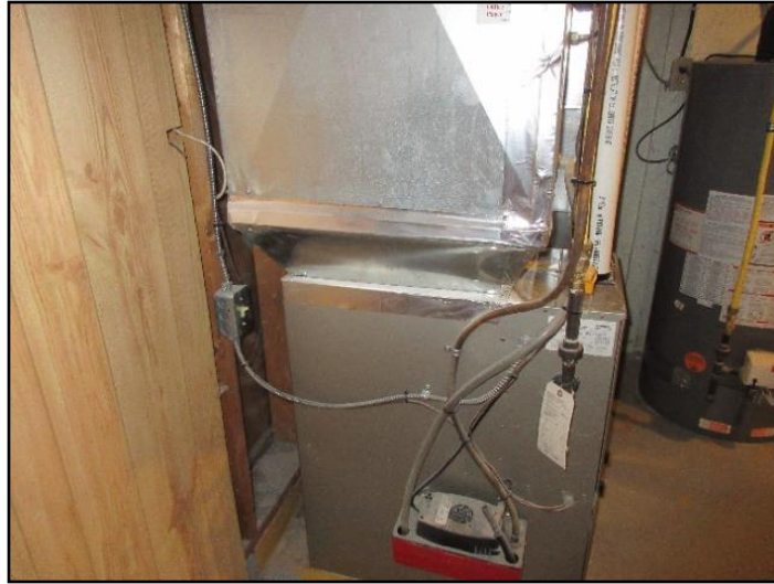
21. Main fuel shut off & electrical disconnect
