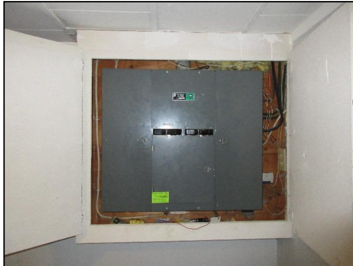
10. Main electrical disconnects
