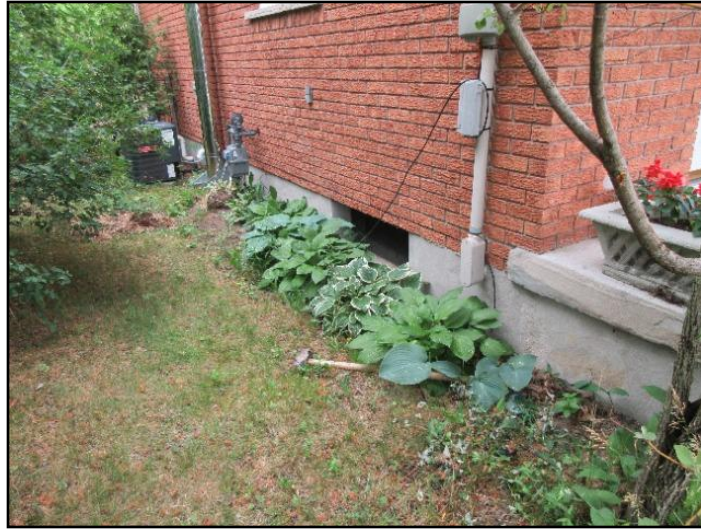
6. Improper slope or drainage
