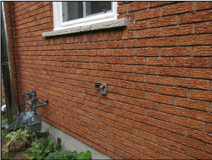
16. No GFCI/GFI (Ground Fault Circuit...)
