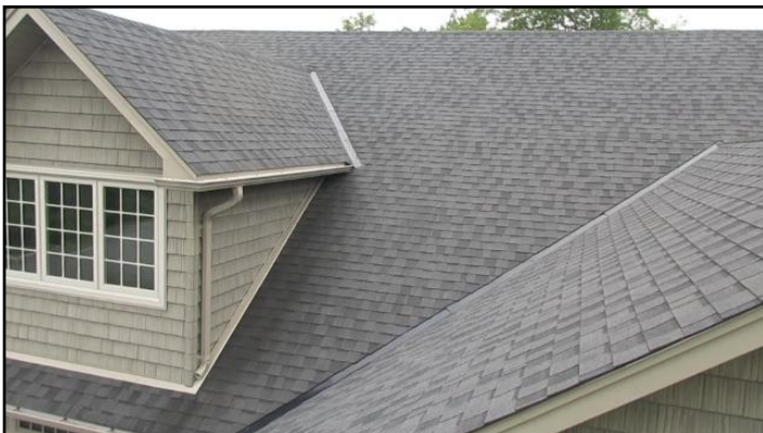
1. Asphalt shingles
