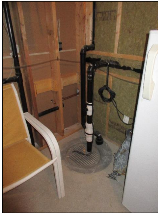
26. Solid waste pump (ejector pump)
