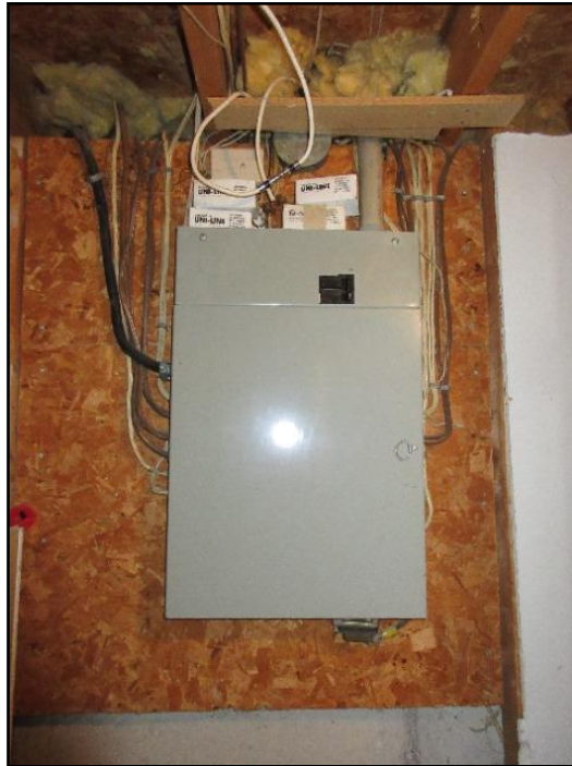
7. Main electrical disconnect
