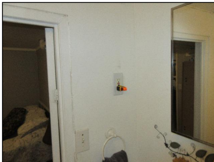
15. Test faulty on GFCI/GFI (Ground Fault...
