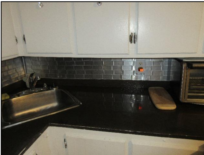
11. No GFCI/GFI (Ground Fault Circuit...
