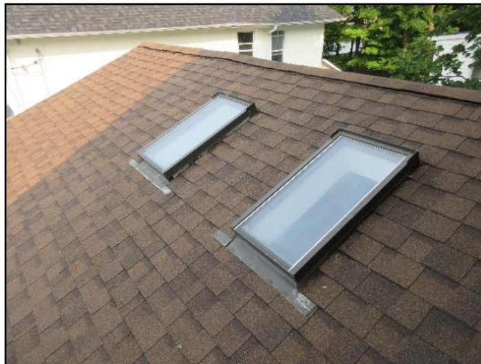
4. Lost seal on double glazing
