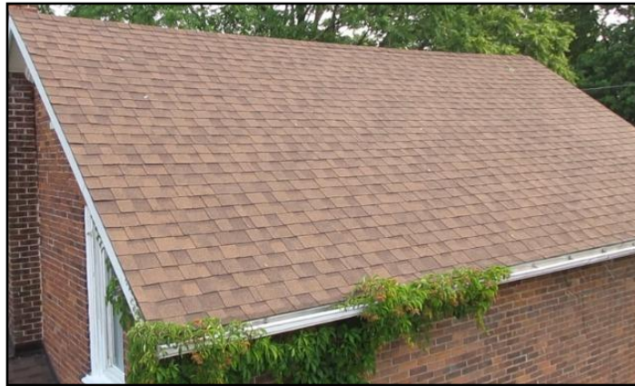
1. Asphalt shingles
