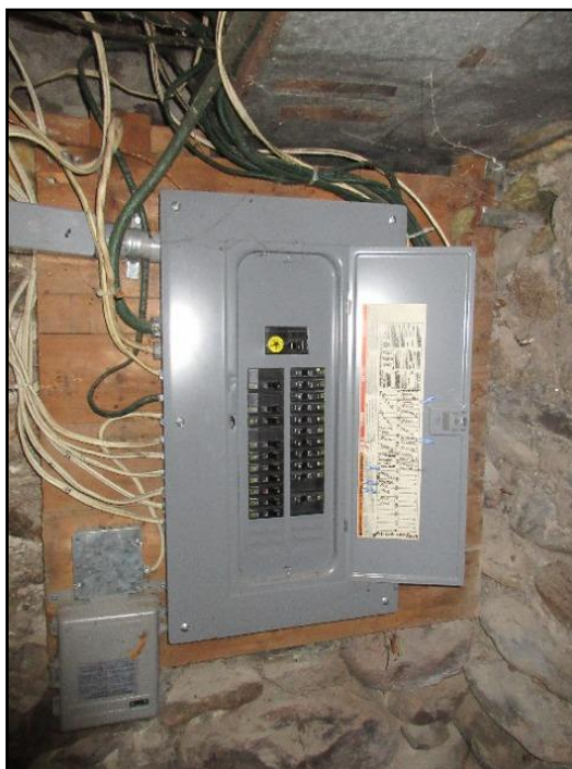
10. Main electrical disconnect
