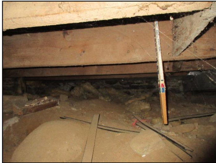
5. Less than 24 inches of vertical clearance...
