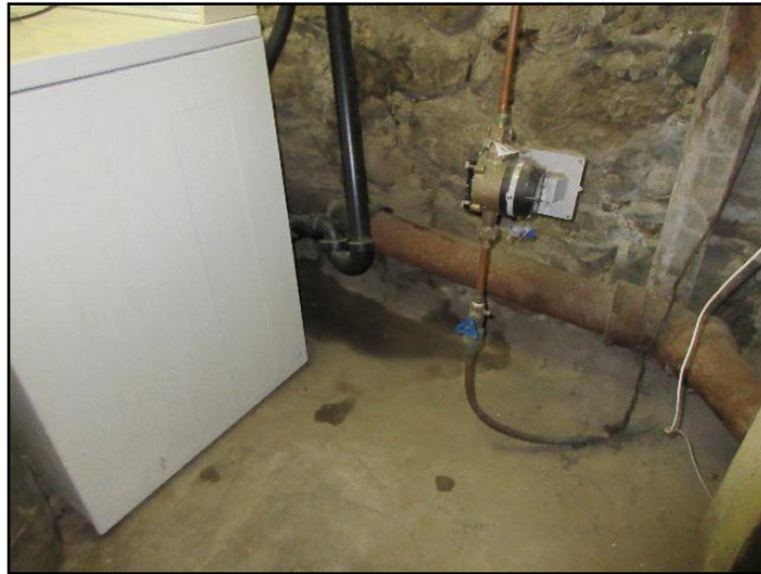
31. Dampness on floor or walls
