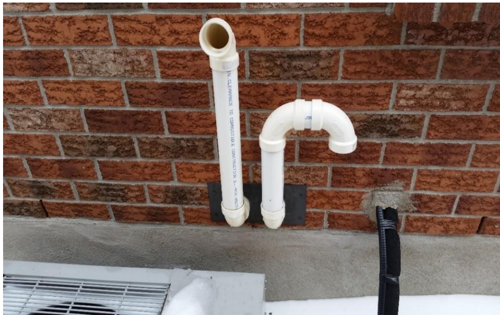
Figure 2.9 - Proper High Efficiency System Intake / Exhaust
