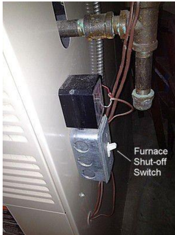
Figure 3.7 - Master Shut-Off or Remote Safety Switch
