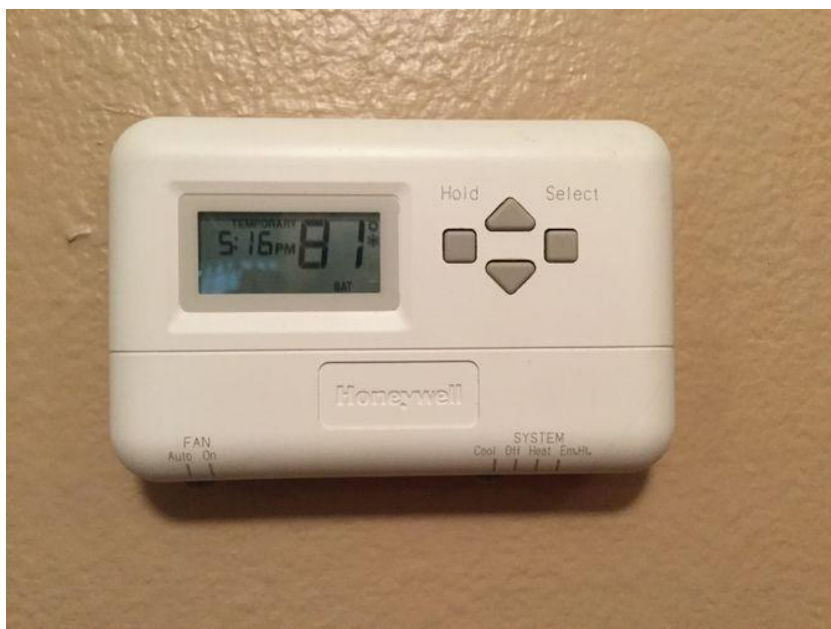
figure 3.4 - Programmable, Digital Clock, Low-Voltage Thermostat
