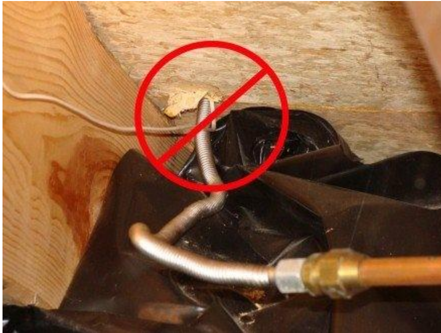
Figure 3.9 - Disappearing Gas Connector
