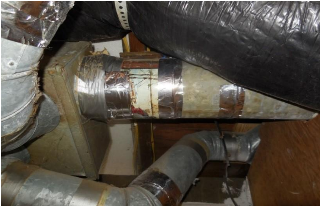
Figure 2.5 - Coffee Can Used to Piece Together a Vent Pipe
