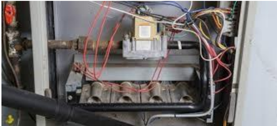
Figure 3.16 - Internals of a Typical Low-Efficiency Gas-Filled System
