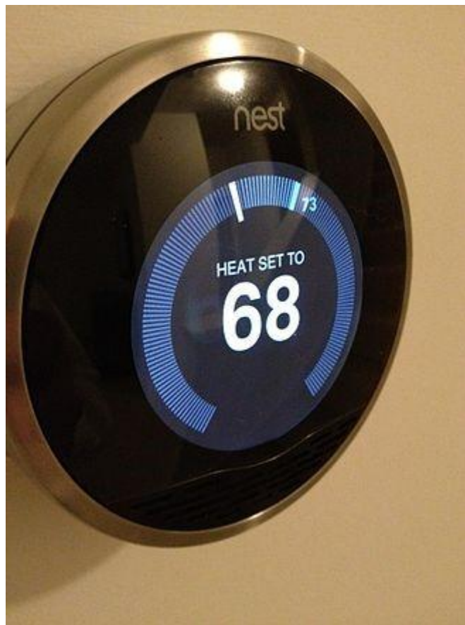
Figure 3.6 - Smart Programmable Thermostat
