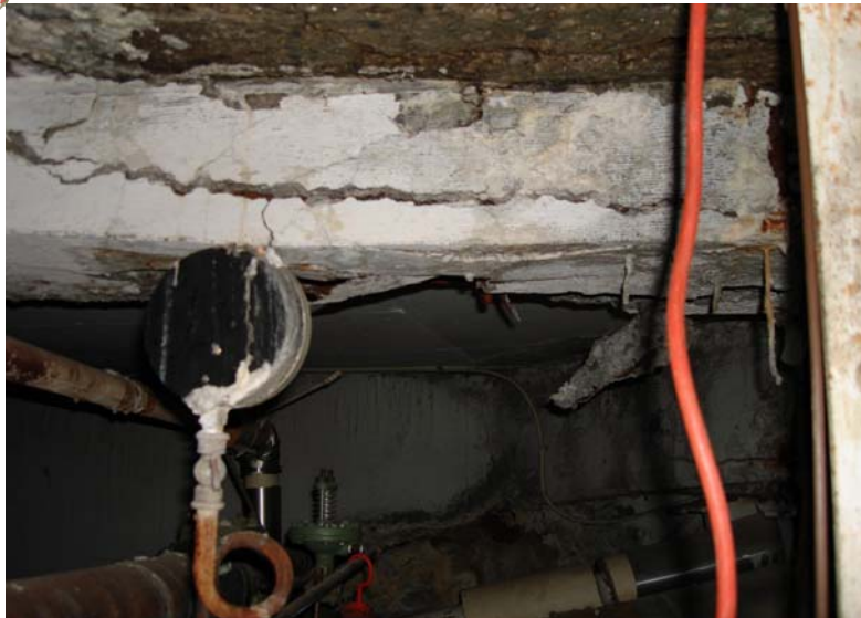
Concrete beam failure
