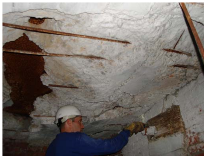
Steam tunnel ceiling collapsed
